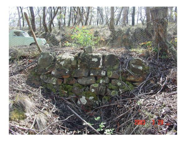
Figure 3.6Remnants of a culvert located on the road as it rises from<br/>the Cox toward Rydal (Solitary Creek) constructed by the<br/>convict iron gangs and road parties in the 1830s. [S.<br/>Rosen, 2003]
